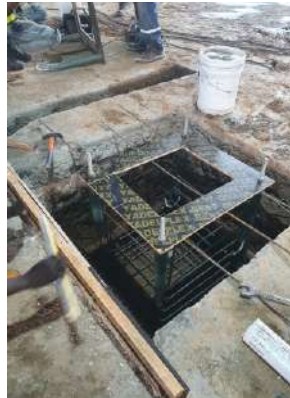
(2022) Machine foundation concrete works for SMC constructions at Nigerite Ikeja
