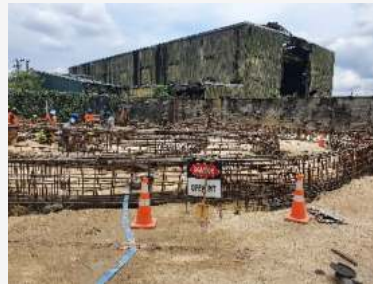
(2021) Structural design & Supervision of foundation for 6000MT bitumen storage tank at NPA, Spar, Port Harcourt
